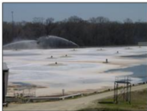
Figure B2. Photo of Conventional Wastewater Treatment via Aerated Stabilization Basin
